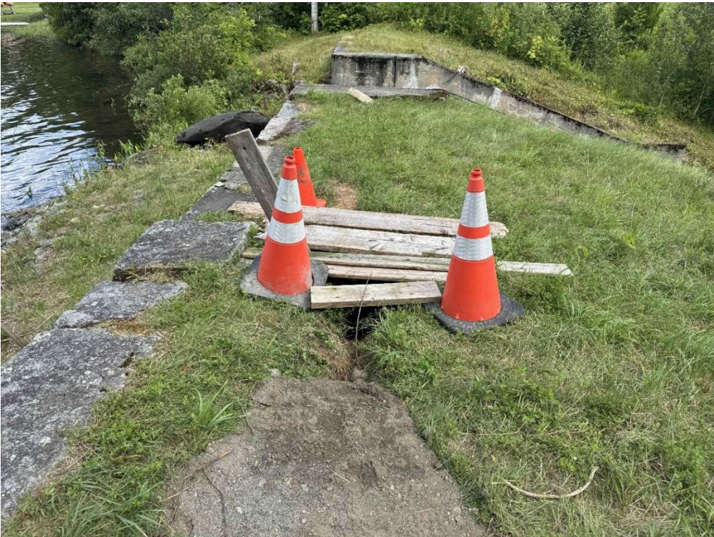
Photo 2: Dam crest, sink hole (looking towards left abutment).
