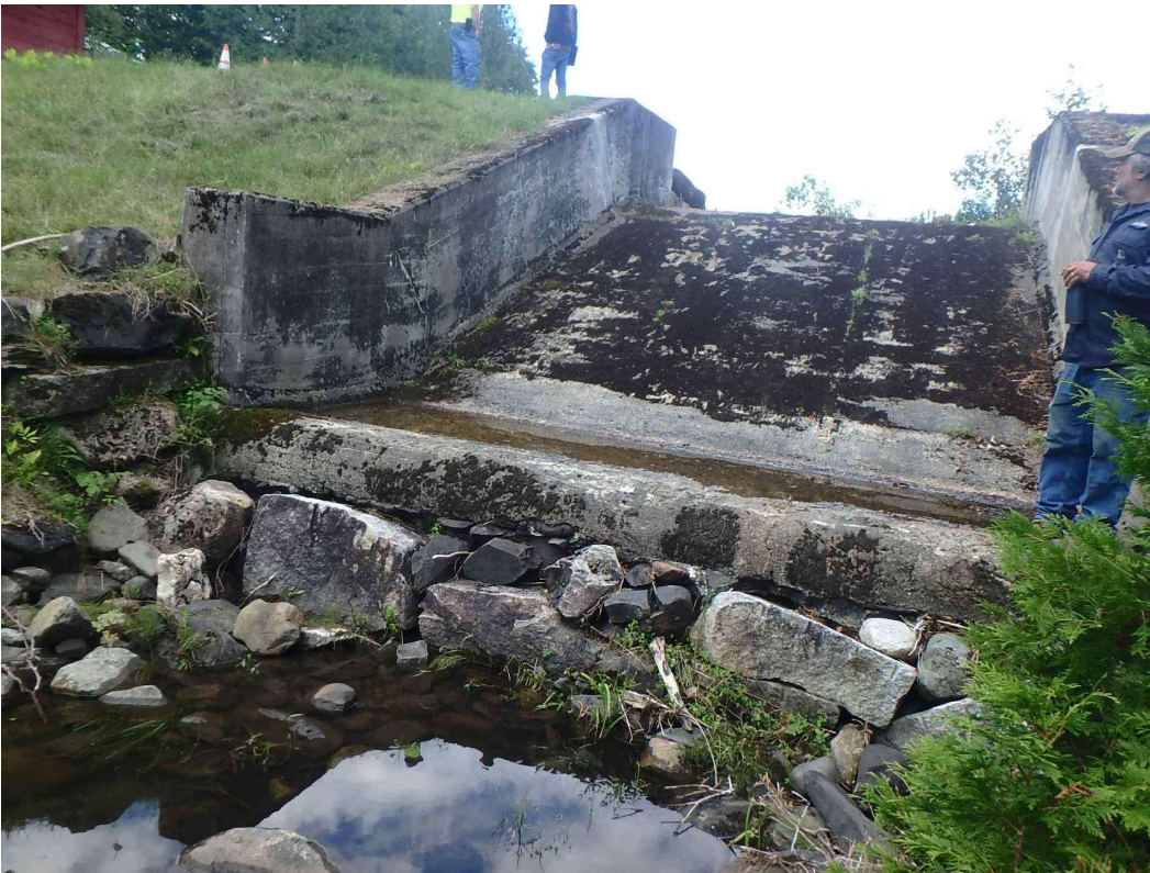
Photo 6: Water pooled below base of auxiliary spillway.
