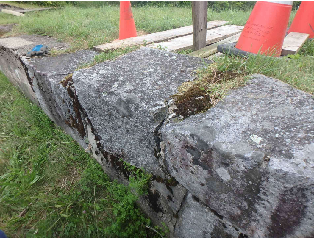
Photo 4: Example masonry blocks and gaps between joints upstream of sinkhole location.
