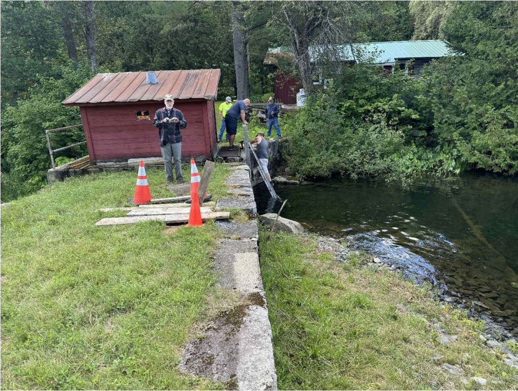
Photo 2: Dam crest, sink hole (looking towards left abutment).
