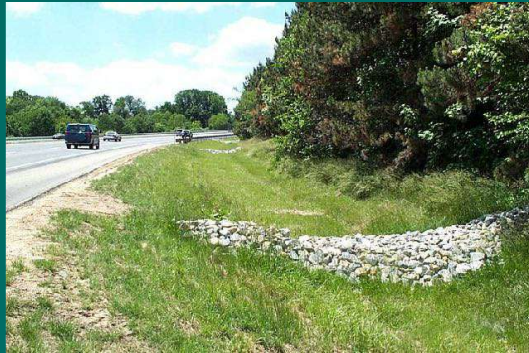
Stone Check Dams
