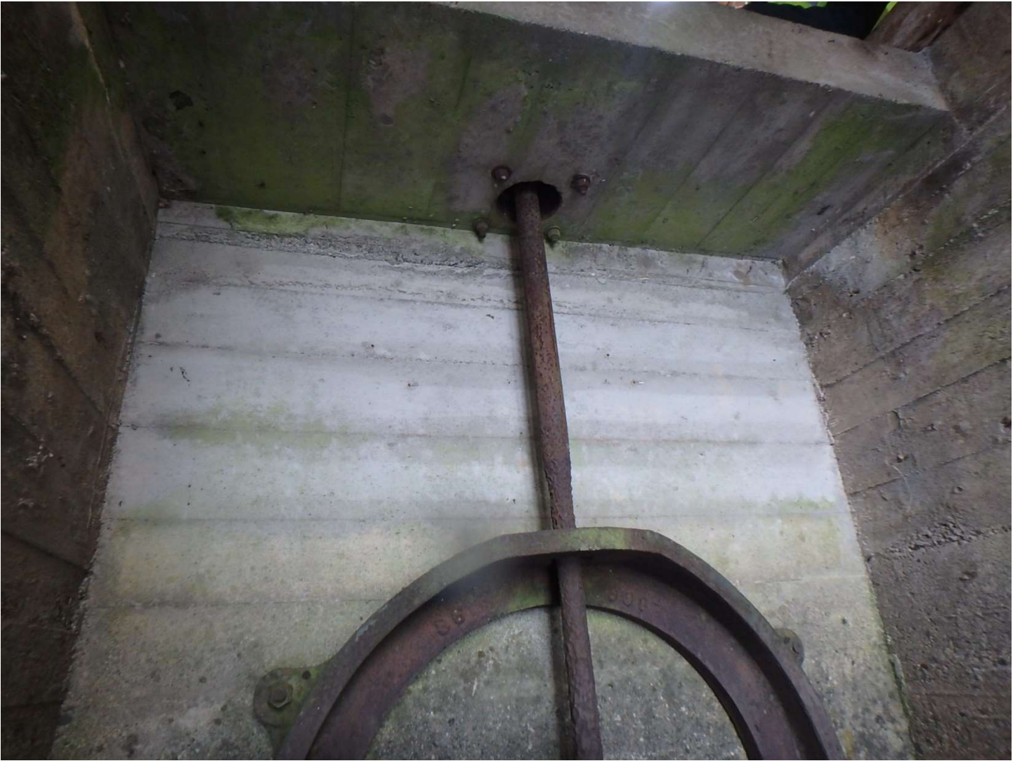
Photo 5: The gate stem where it enters the floor, above.
