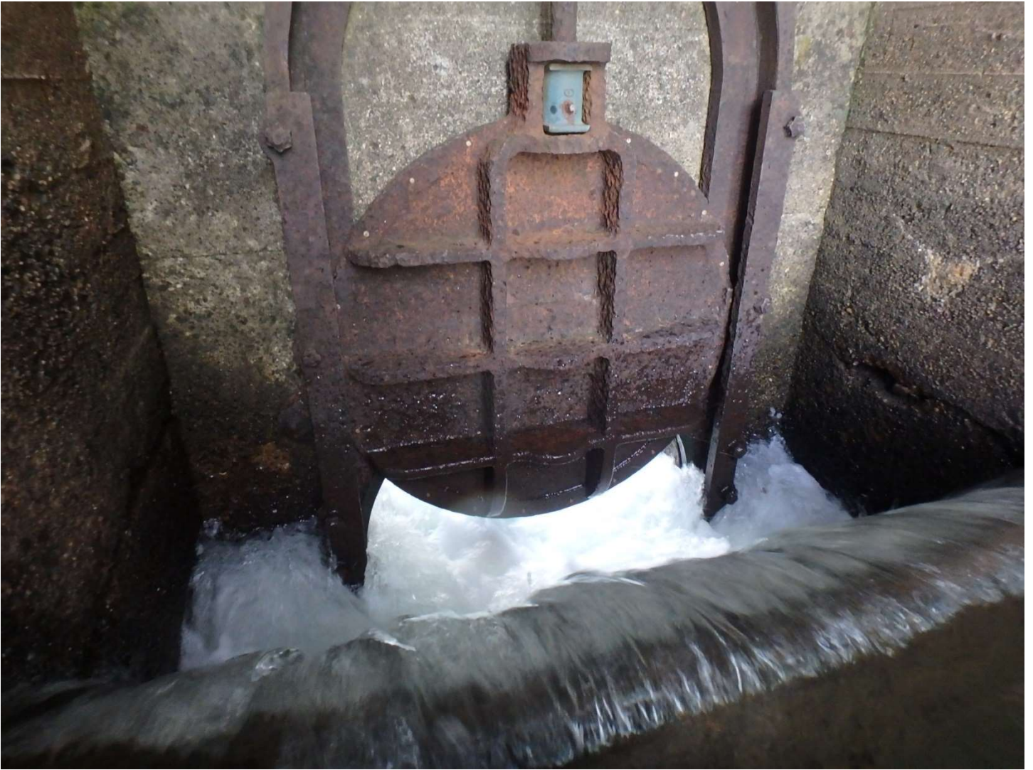
Photo 4: The gate downstream of the stoplogs looking downstream.
